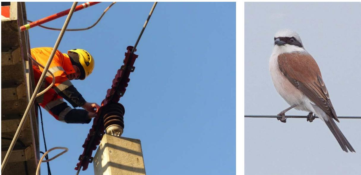
*Figure 28: Measures to reduce the number of these short circuits - application of a guard-device in front of the insulator and a bird protection cap on top of the catenary pole (left) Lanius collurio (right) © ÖBB - Infra*
