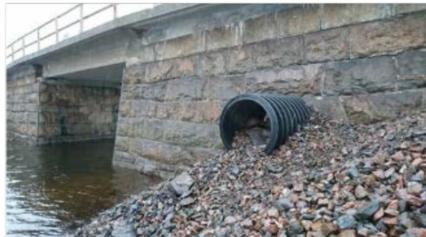
*Figure 15: Pipes and ducts to facilitate movement of medium-sized mammals under Swedish railways, © Trafikverket*
